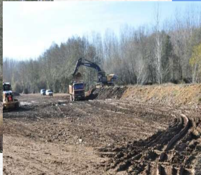
Rest of levee after removal and setback in an urban stretch wich remains as an example
